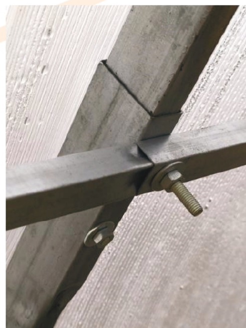
Figure 6 - View of the interposition of the arcs and crossbeams when they are connected
